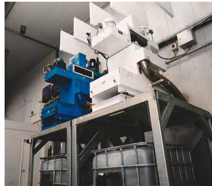
Micro separators at Budweg's plant in Denmark cleaning recycled water
